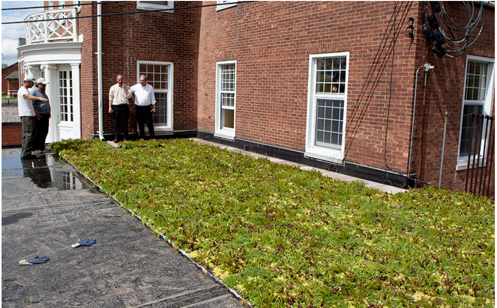
Buildings and Grounds staff meet with contractors who are installing a green roof on Comstock Hall. The pilot project was initiated by the Climate task force as a means to help with storm water management, reduce the heat island effect, and improve the insulation in the new Comstock renovation. (2011)
