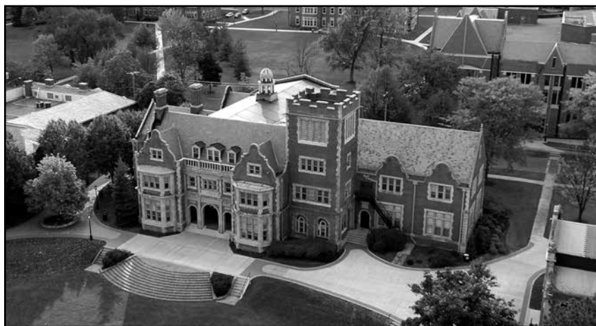
Aerial view of the campus, ca. 2005
