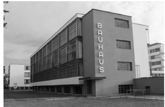
Bauhaus Building in Dessau
