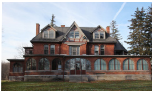
Houghton House (1880) 1 King's Lane
