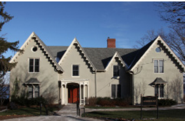
Bradford House (1840) 629 South Main
